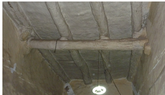
Figure 7. Interaction between floor beams and adobe walls for C.A.
